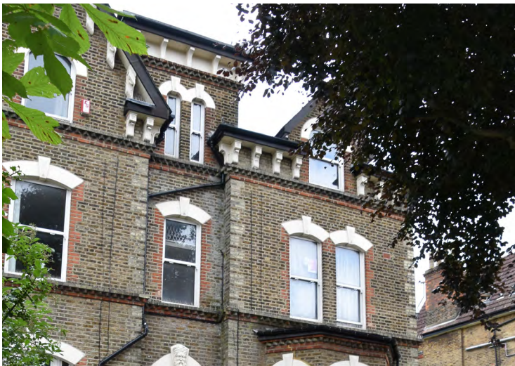
65. Example of London stock brick, red brick and stucco detailing on Warminster Road
