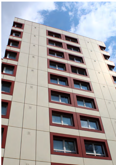
44. Late 1960s tower block on Belgrave Road
