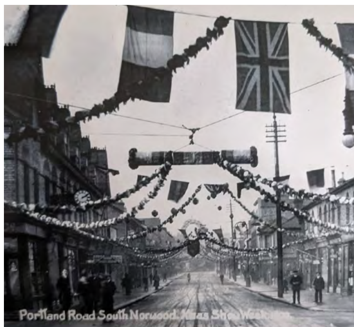
38. Decorations along Portland Road, South Norwood (source: James Bentley Archives)
