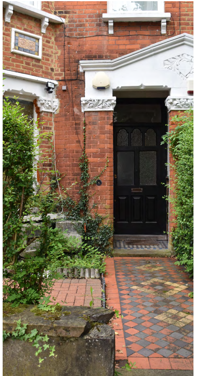
66. Residential building on Chalfont Road, demonstrating well preserved historic architectural detailing and tiled entrance
