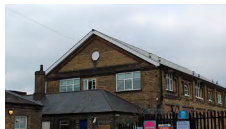
8. The goods shed at Norwood Junction Station
