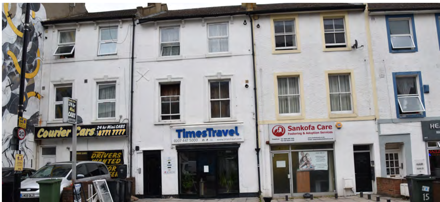
145. Example of loss of traditional windows on buildings on the left hand side and right hand side
