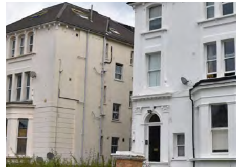
91. Painted render with sash windows
