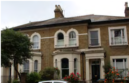
86. London stock brick, stucco, and slate roofing
