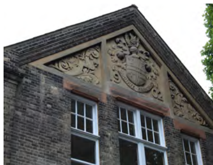
89. London stock brick and carved stone detailing (Samuel Coleridge-Taylor Centre)
