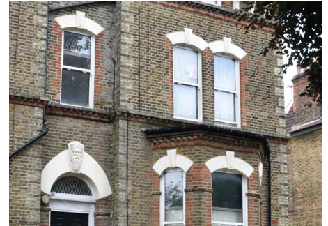
82.Keystones over arched windows and entrance
