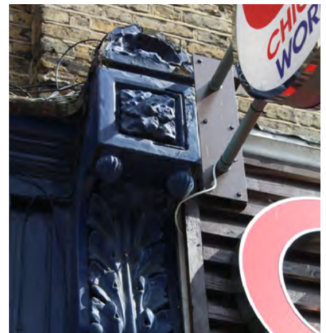
83.Historic shopfront detail
