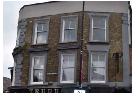
90. Timber sash windows
