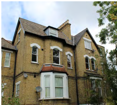
116. No. 2-2D Lancaster Road, a prominent corner plot building
