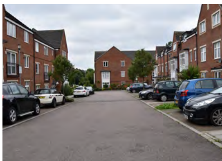
14.Recent residential development on Chalfont Road
