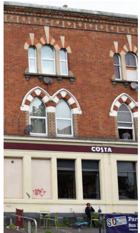
95.Nos. 249 - 251 Selhurst Road
