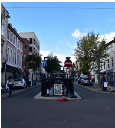
98. View north along Station Road
