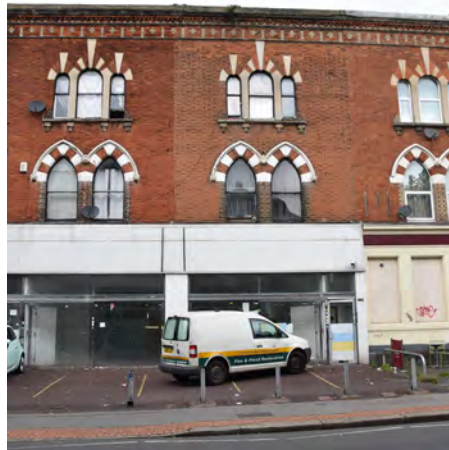
148. Example of a vacant building within the Conservation Area
