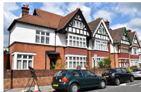
11. Semi-detached houses on Albert Road
